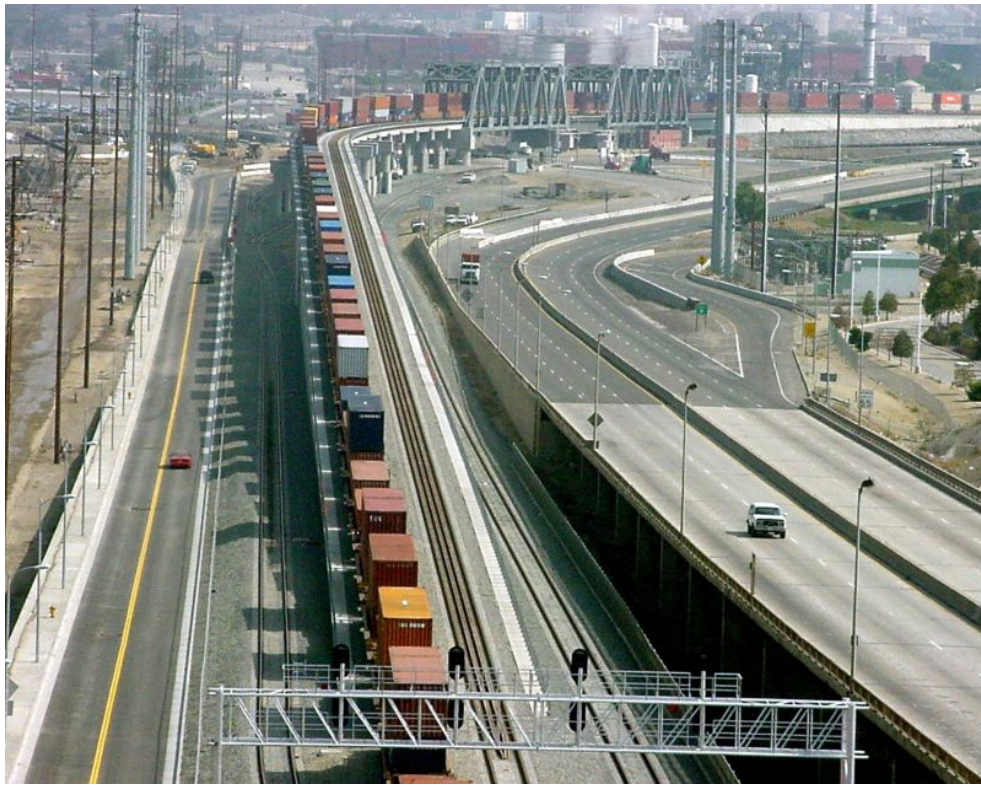
FIGURE 8: DOUBLE STACKED TRAIN ON THE ALAMEDA CORRIDOR
