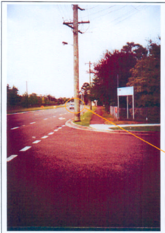
This is an example of a power pole restricting the view of the traffic. The photograph was taken from the driving position of a car turning right at Lewin Street, Springwood. Behind the power pole is another car almost completely blocked from view.
