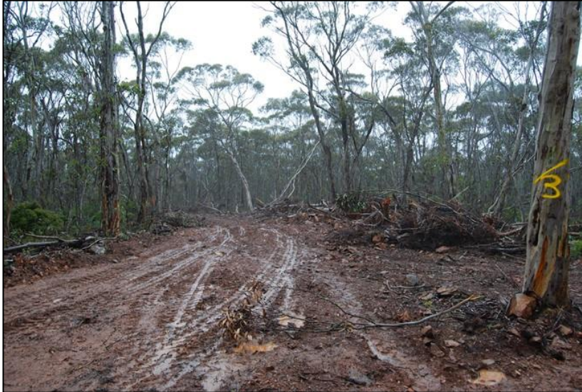
Plate 2-1: Road construction – track recently widened and drained
