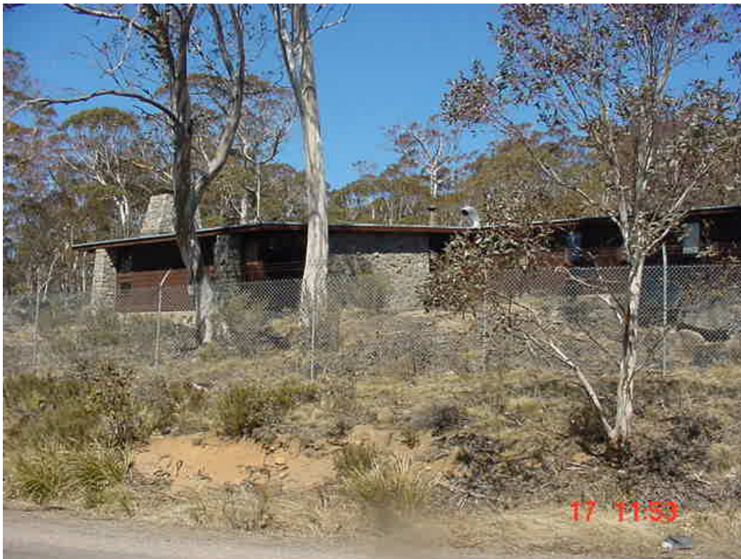
PHOTOGRAPH No.45. RTA Workshop and living quarters (near Wilson's Creek)
