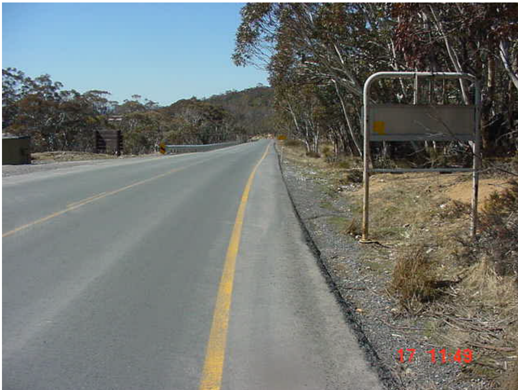
PHOTOGRAPH No.43. Kosciuszko Road -sealed shoulder (with runoff gutter)
