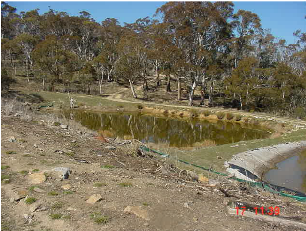
PHOTOGRAPH No.40. Secondary settling pond (unlined)
