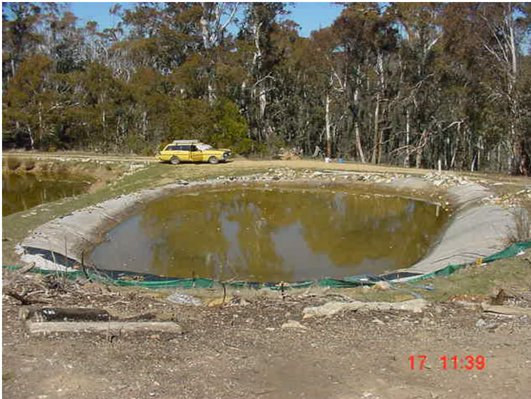
PHOTOGRAPH No.39. Leachate primary settling pond (plastic lined)
