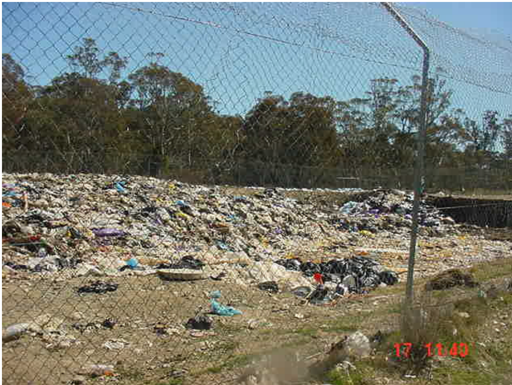
PHOTOGRAPH No.41. Current landfill – no evidence of daily soil cover
