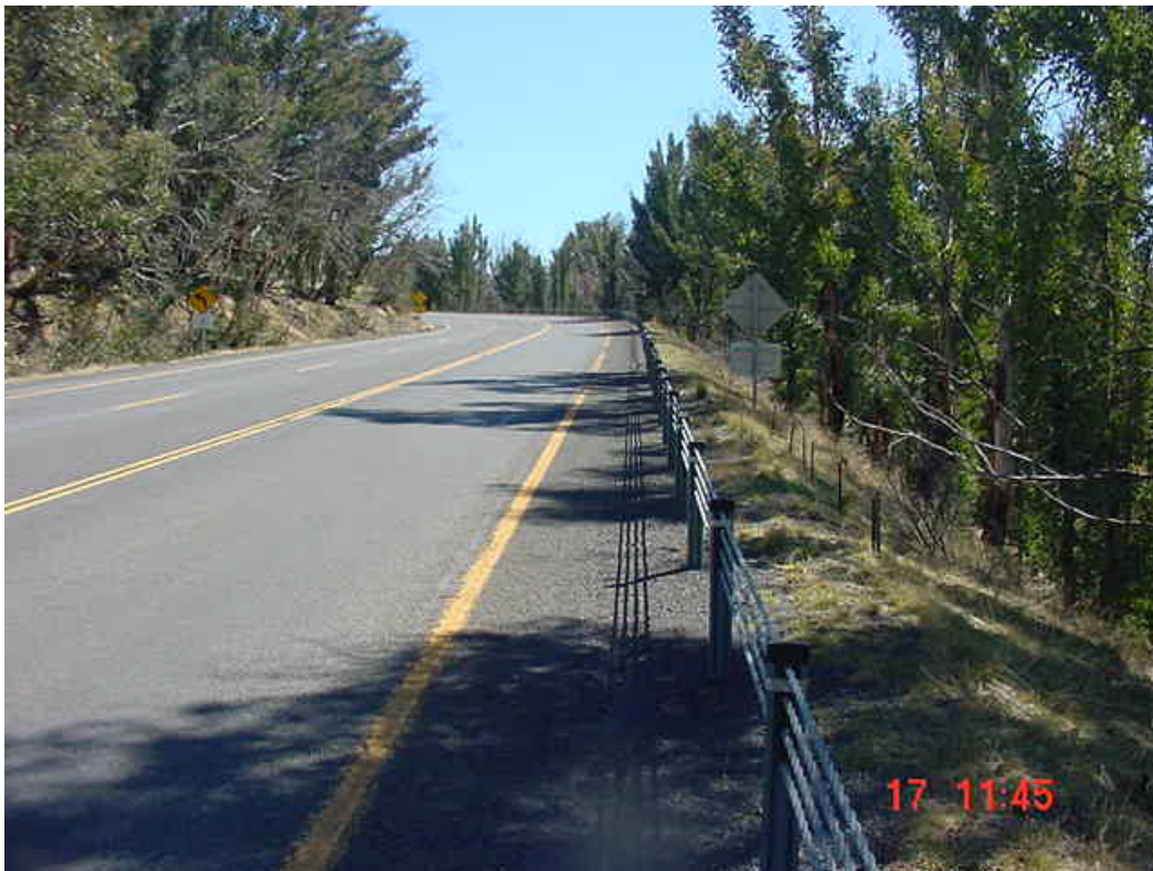
PHOTOGRAPH No.42. Kosciuszko Road (good section – sealed to edge & fenced.
