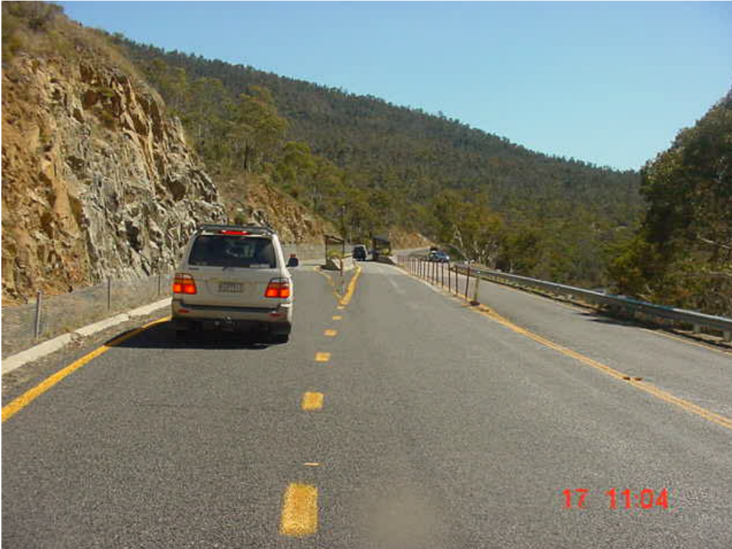
PHOTOGRAPH No.29. Gate entry / Exit on Kosciuszko Road
