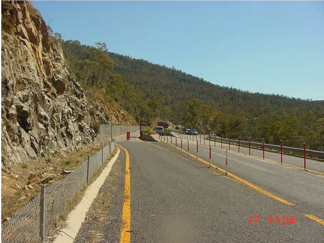
PHOTOGRAPH No.27. Gate entry to KNP on Kosciuszko Road
