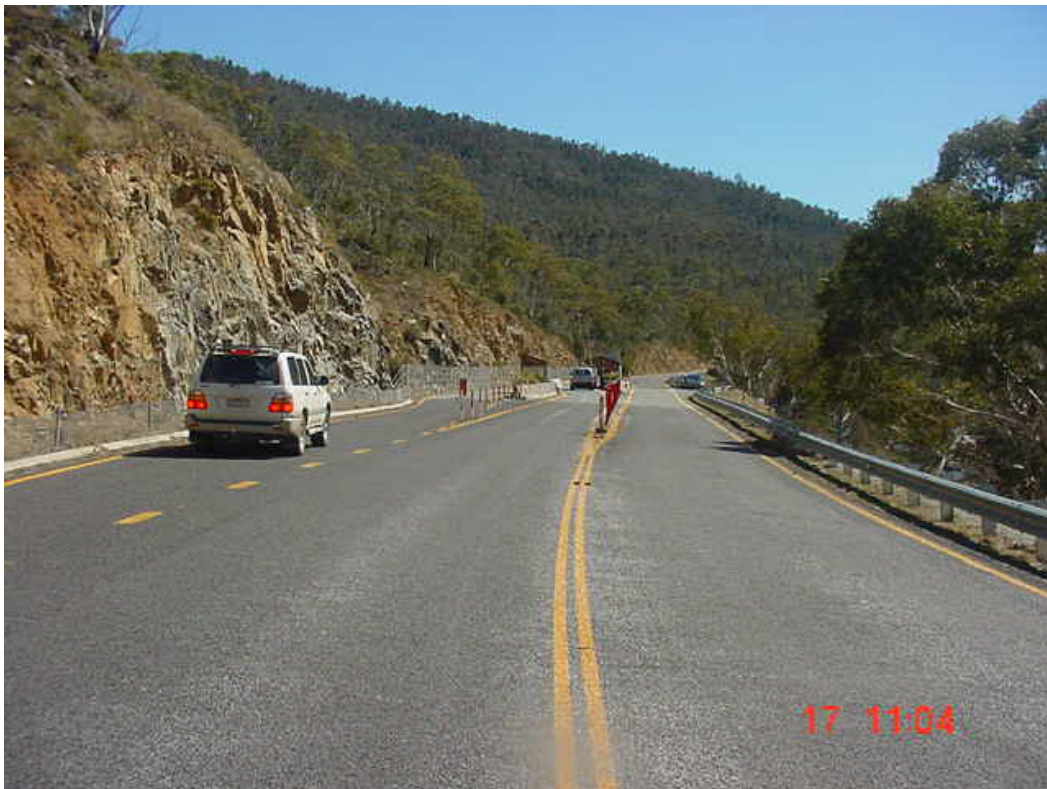
PHOTOGRAPH No.28. Gate entry / exit on Kosciuszko Road
