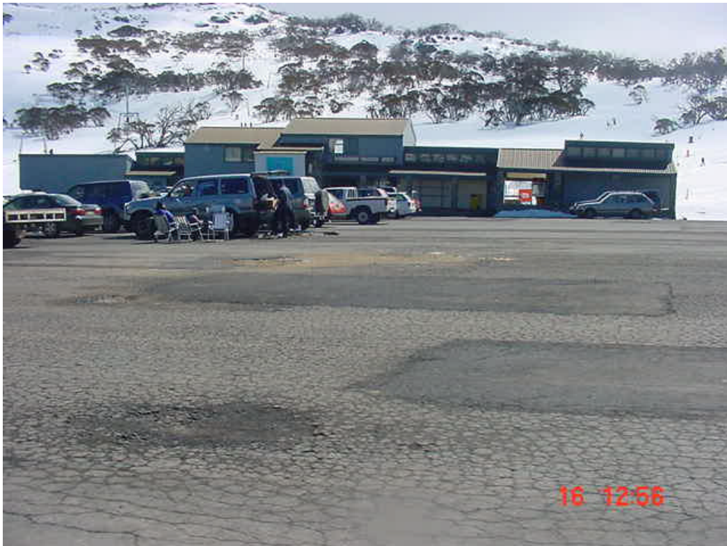
PHOTOGRAPH No.25. Car park condition at Smiggin Holes (looking toward workshop)
