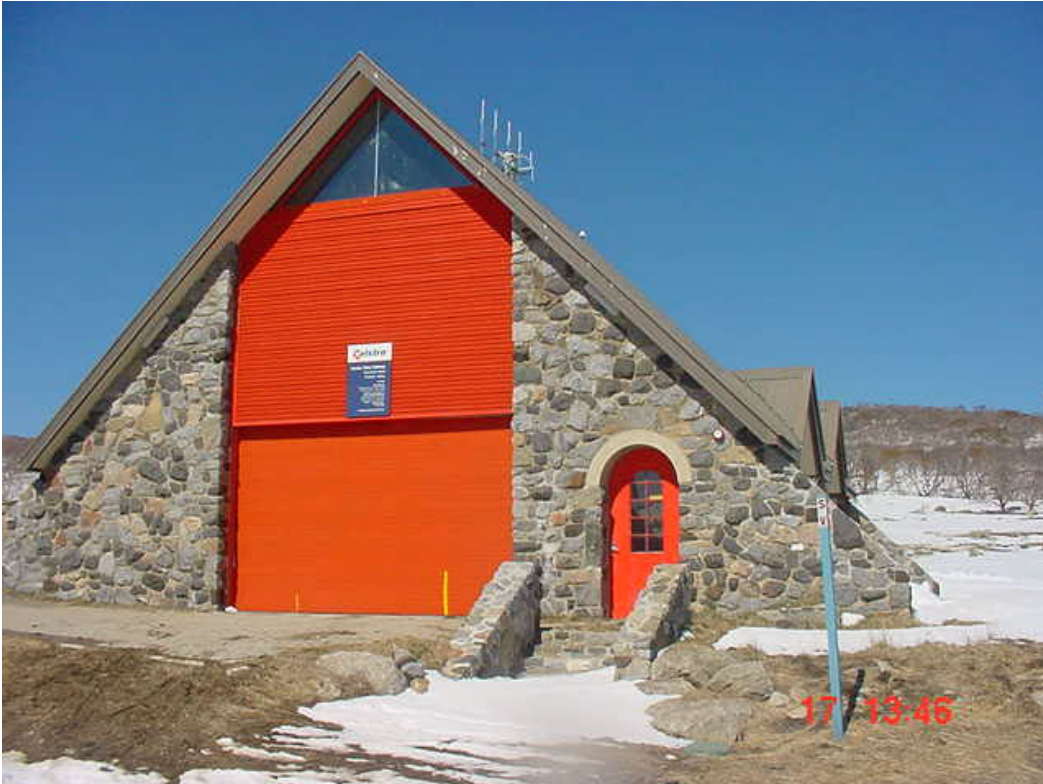
PHOTOGRAPH No.13. Communication Station
