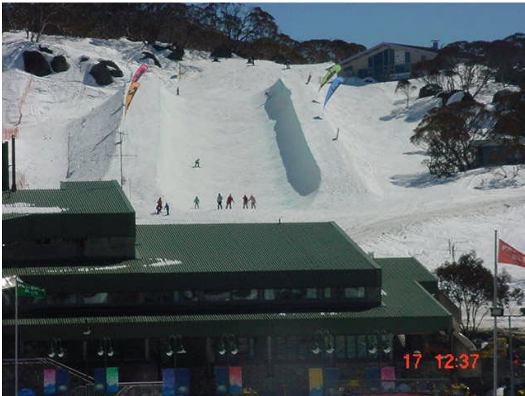
PHOTOGRAPH No.4. View from Workshop over PBL Building to Super Pipe
