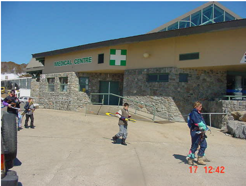
PHOTOGRAPH No.6. Medical Centre (at North end of Ski tube terminal)
