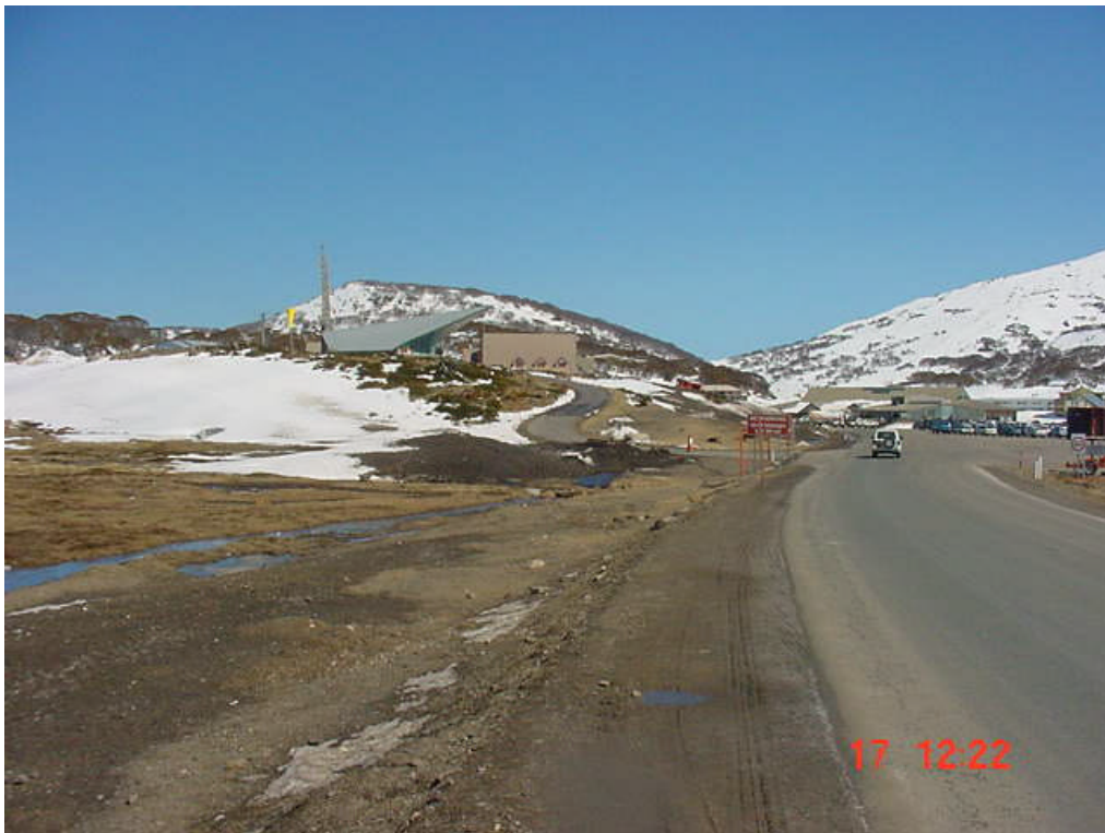
PHOTOGRAPH No.1. Main Entrance to Perisher – gravel shoulders
