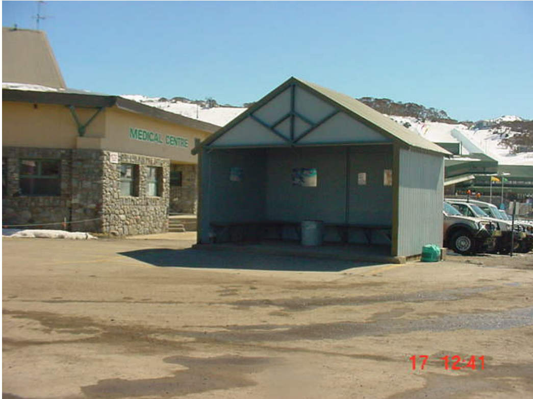
PHOTOGRAPH No.5. Shuttle Bus stop alongside Ski tube terminal
