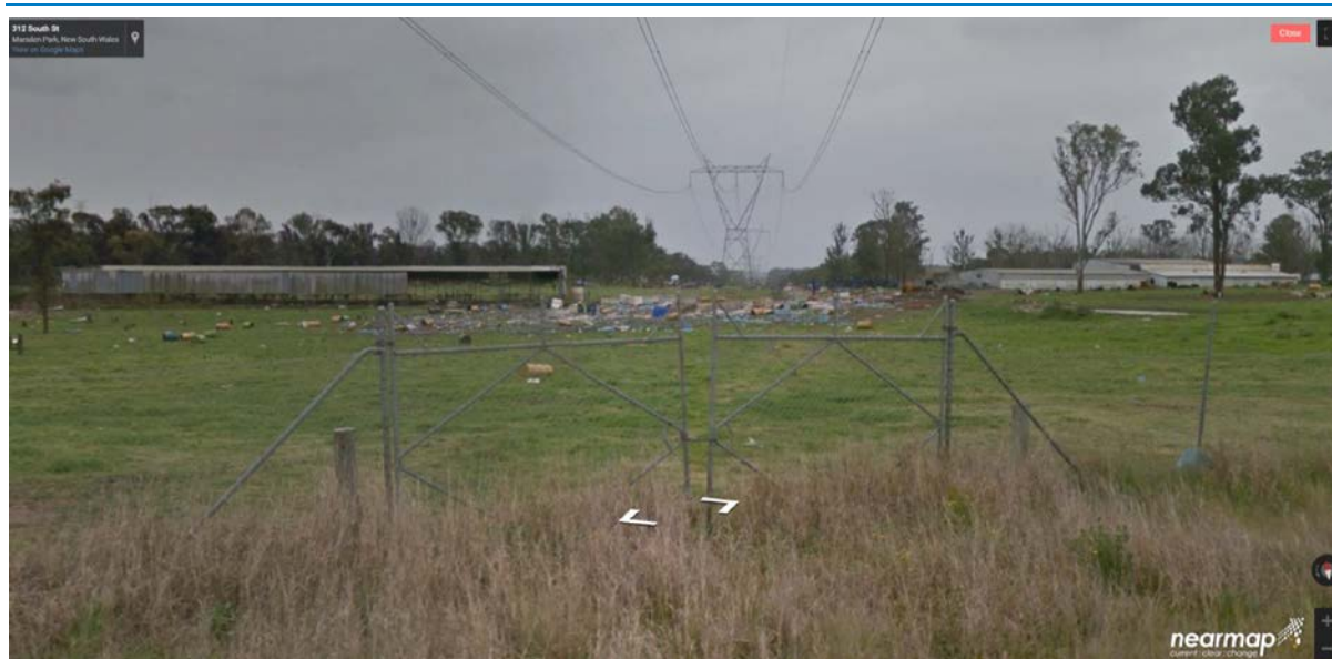
Figure 4.2 Example of open space land requiring site preparation – Reserve 992
