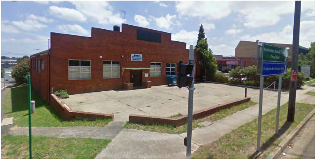
Figure 4: Existing light industrial building at No. 2 Constitution Road (Source: Google Maps)
