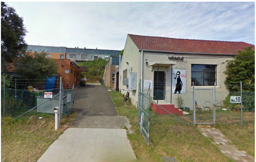
Figure 5: Former light industrial building fronting Rothesay Avenue (Source: Google Maps)
