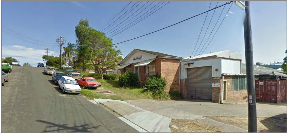
Figure 6: Former light industrial building fronting Nancarrow Avenue (Source: Google Maps)
