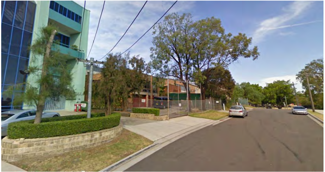
Figure 4: Former light industrial building fronting Rothesay Avenue (Source: Google Maps)
