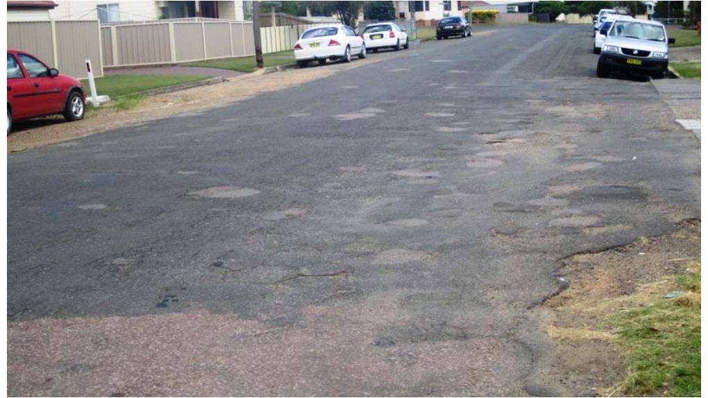
Very Poor – PCI Range between 1.0 and 2.49
