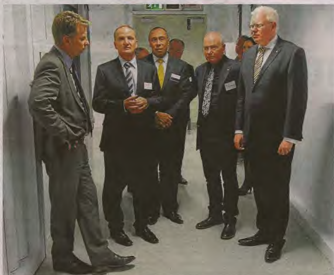
Official visit: Touring the Unanderra centre that provides back-up for NSW government information are Finance Minister Andrew Constance, NextGen chief executive Peter McGrath, Metronode general manager Malcolm Roe, Wollongong Lord Mayor Gordon Bradbery and Kiama MP Gareth Ward. PICTURE: GREG TOTMAN
