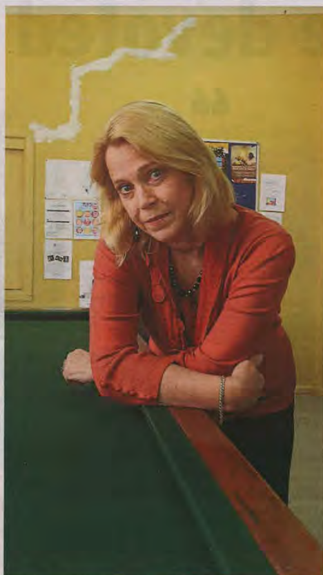
Cracks in walls: Wollongong City Council's Jan Noble says Berkeley residents will have to make hard decisions over the future of the run-down Berkeley Neighbourhood Centre. Picture: ROBERT PEET
