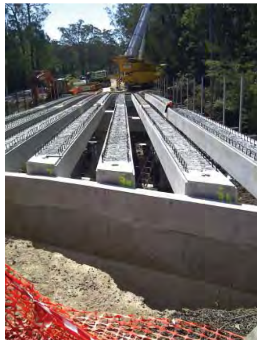
The Booral Creek bridge works.
