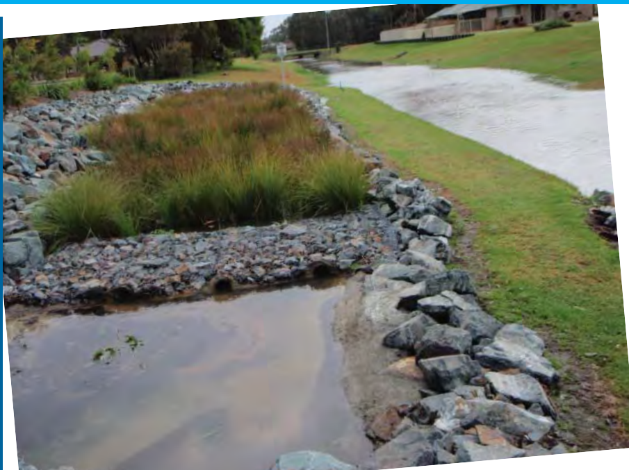
The Levy helps fund the construction of water quality gardens and wetlands in urban areas to treat stormwater runoff.
