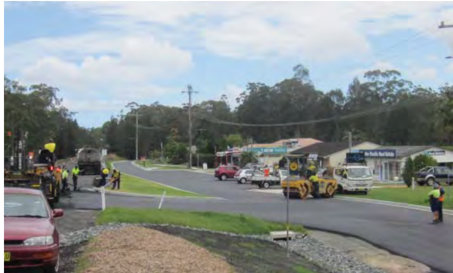
The Lakes Way and Charlotte Street reconstruction has recently been completed.
