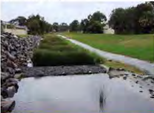
The ESR has enabled the construction of water quality gardens. The gardens improve water quality in Wallis Lake by filtering urban run-off.
