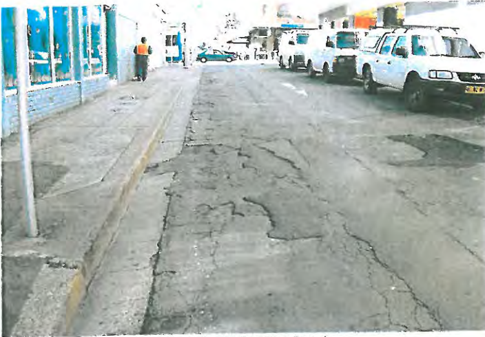
Example of a Condition 5 road
