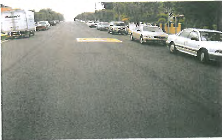
Example of a Condition 1 road
