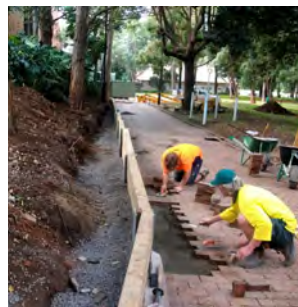
Road and Footpath Upgrade
