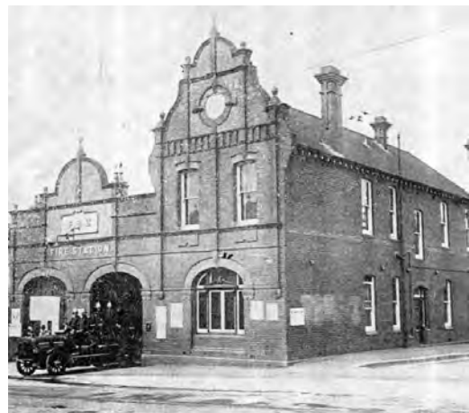
Burwood Fire Station (1900-1925) Cnr Belmore Street and Burwood Road, Burwood
