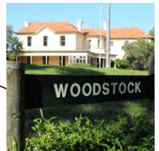
Woodstock Community Centre Upgrade
