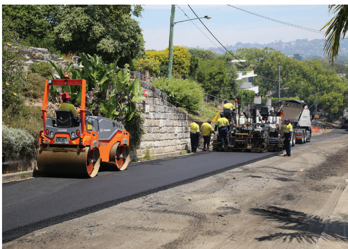
Road re-surfacing works
