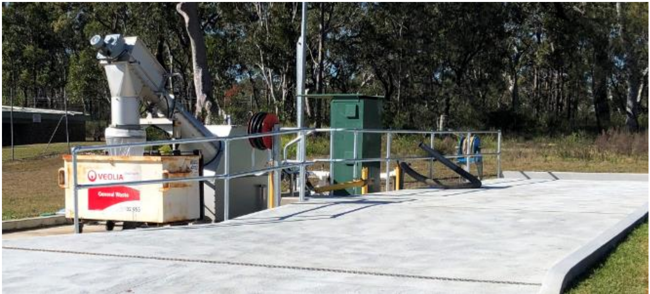
Figure 3: Septic receiving station allows for safe discharge of tankered septic waste, measurement of discharge volumes and rag removal
