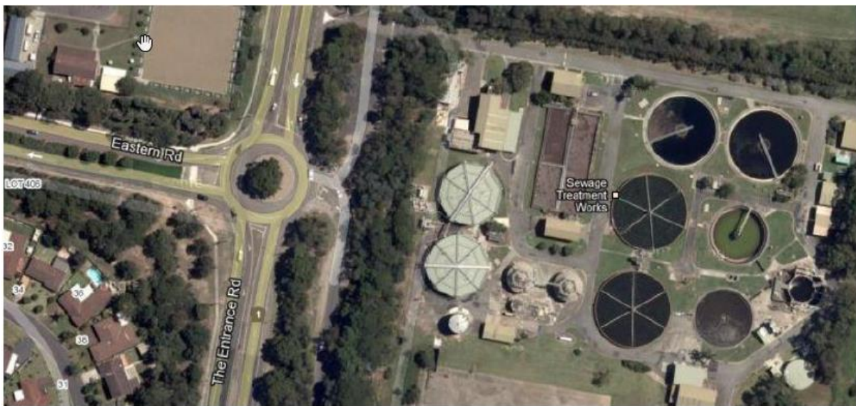
Figure 43: Bateau Bay sewage treatment plant aerial view
