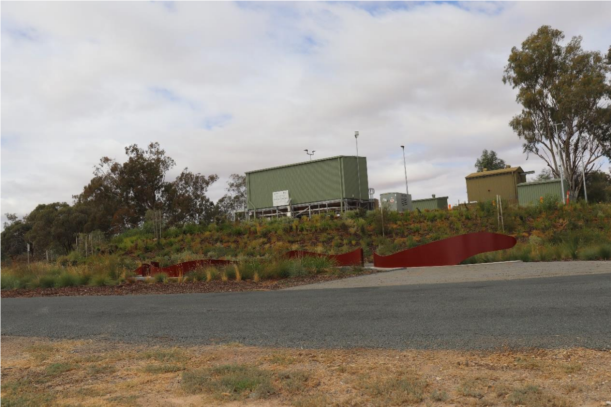
Figure 11 - The River Murray Pump Station
