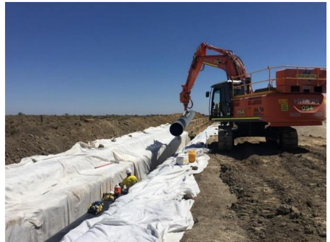
Figure 27 - Machine laying pipe
