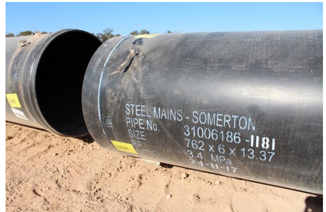
Figure 30 - Picture of pipe during stringing process
