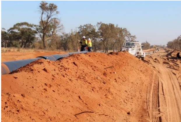
Figure 28 - Pipe strung at the southern end of the pipeline route
