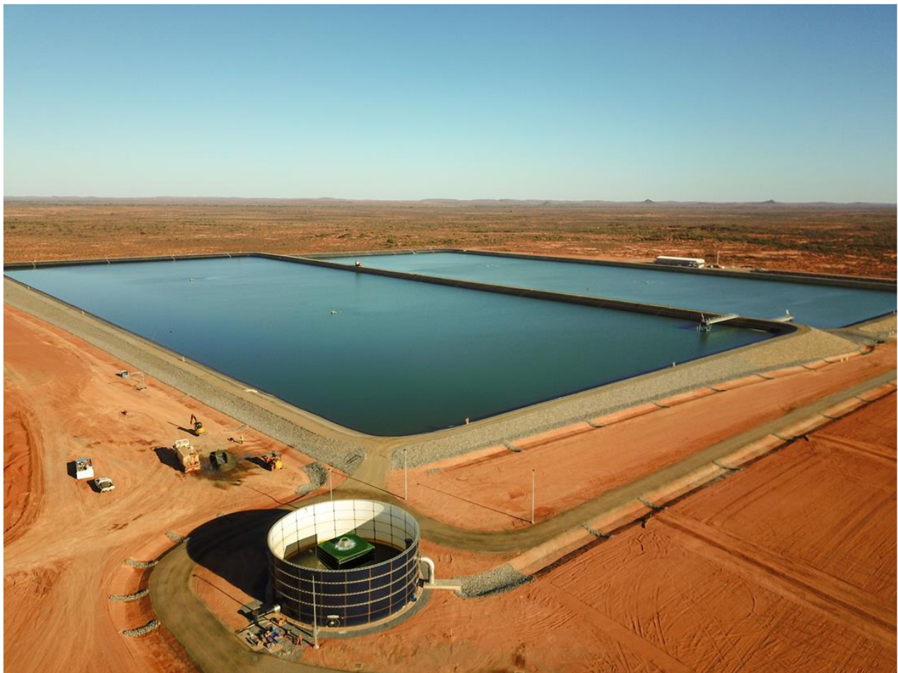
Figure 5 - WaterNSW’s bulk water storage facility
