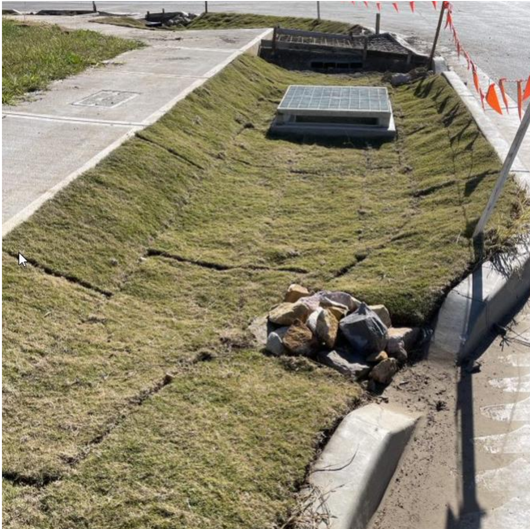
Figure 2 - Newly Constructed Raingarden (silt trap phase - pre-raingarden)
