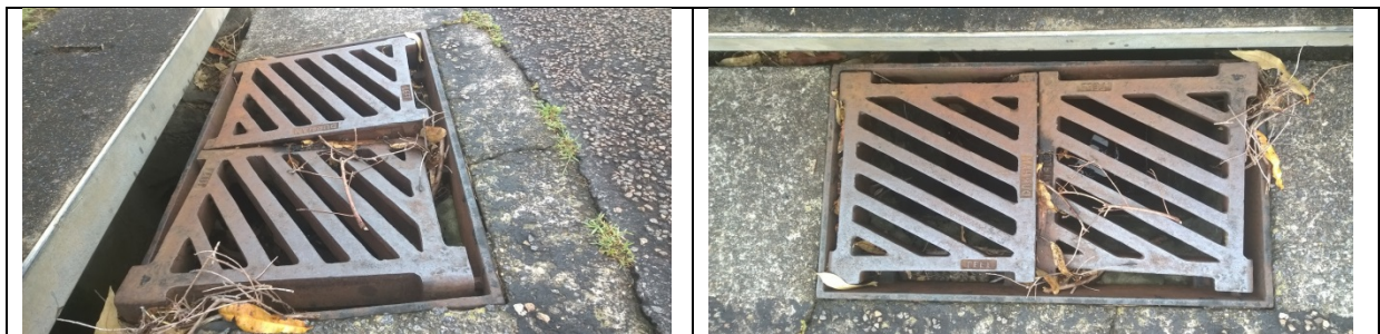
Stormwater drain up from Fairchild Street Raymond Terrace
