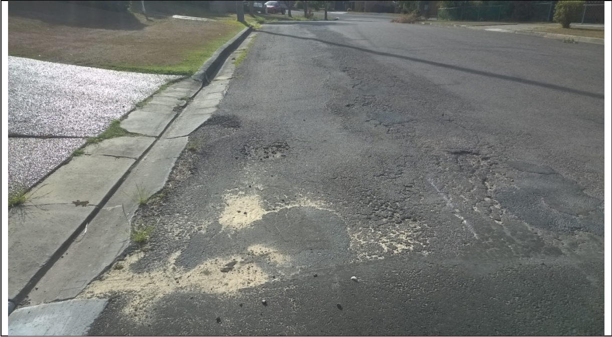
Pennington Road end of new section and joint with old.
