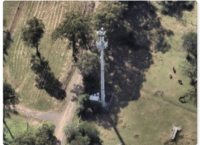
Elevation view of facility:
