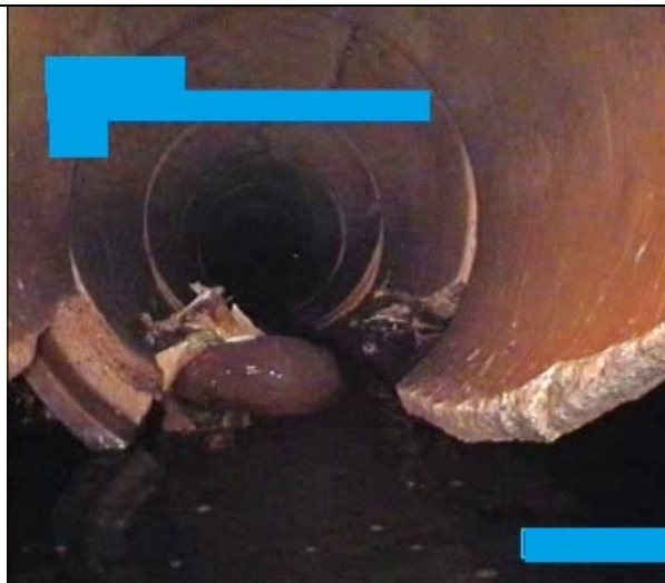
Stormwater Pipes in very poor condition – collapsed
