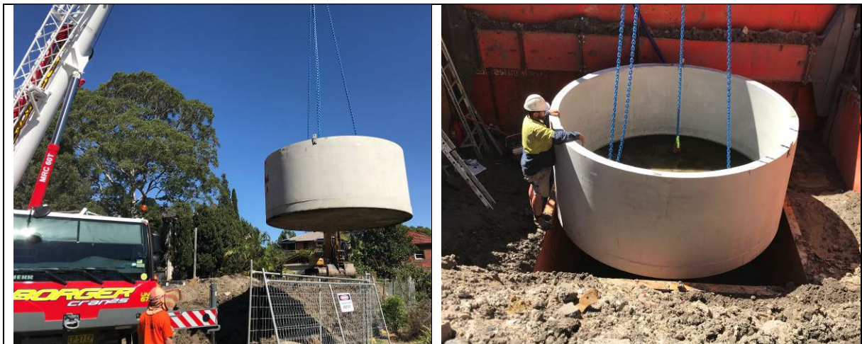
Replacement of GPT at Little Young Street, Cremorne.
