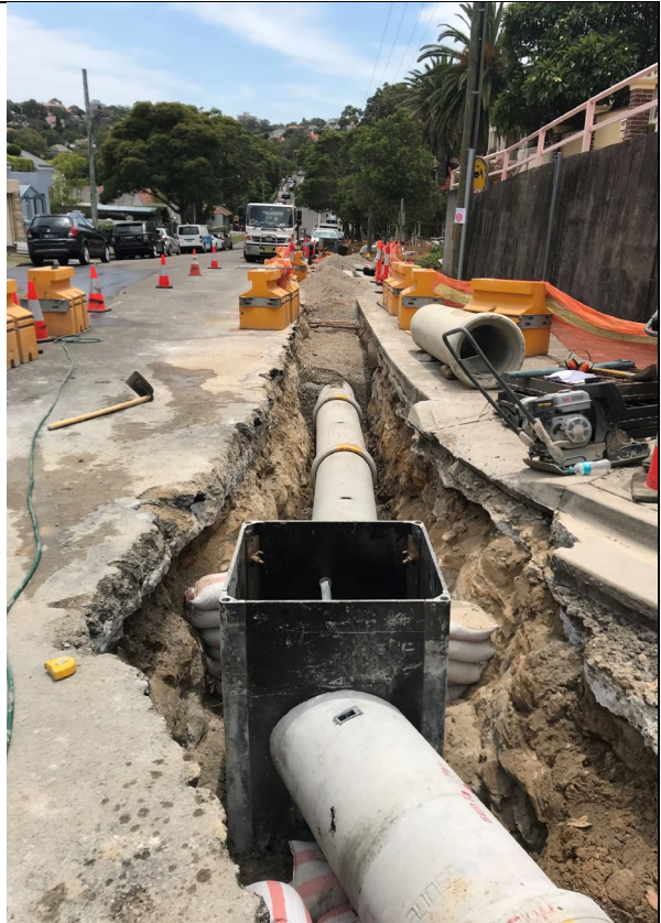
Pit and Pipe replacement at Milson Road, Cremorne Point.
