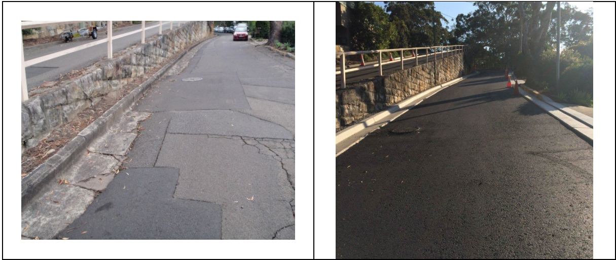
Road Pavement - Folly Point, Cammeray, before and after
