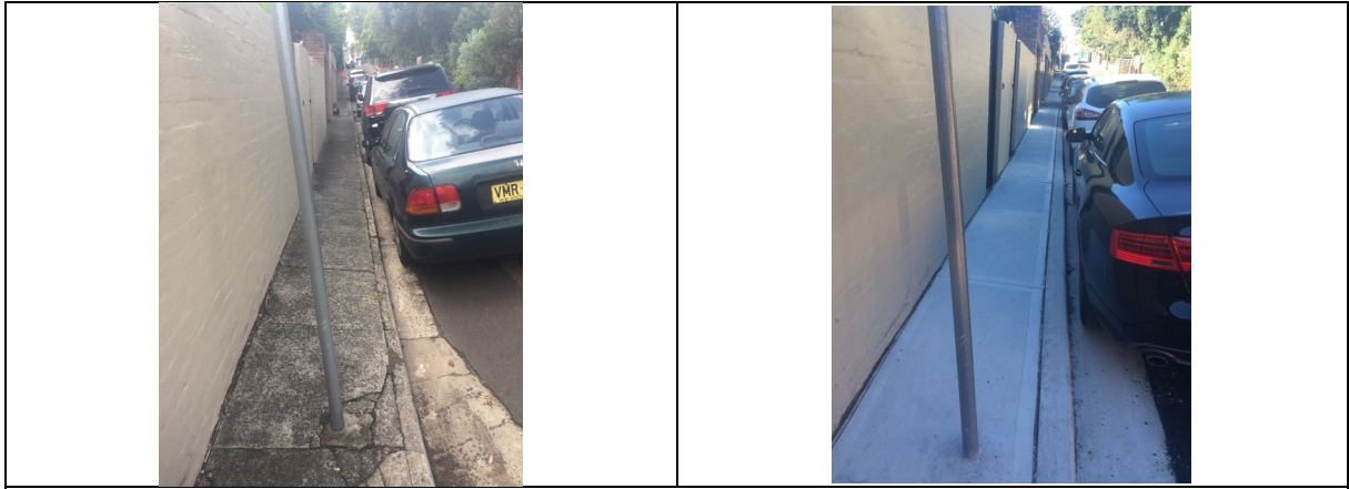
Kerb and Gutter, Crescent Place, Kirribilli – Before and After
