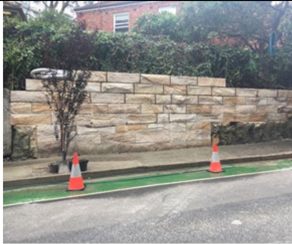
Retaining Wall - Middlemiss Street, North Sydney
