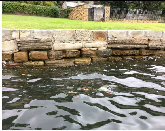
Seawall Grout Injection rehabilitation at Sawmillers Reserve -- before
