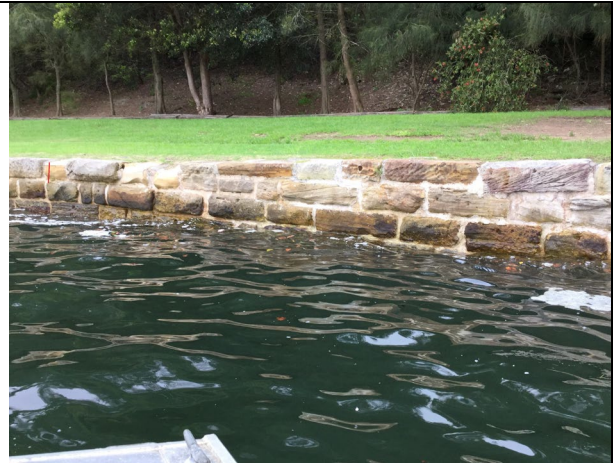
Seawall Grout Injection rehabilitation at Sawmillers Reserve -- after
