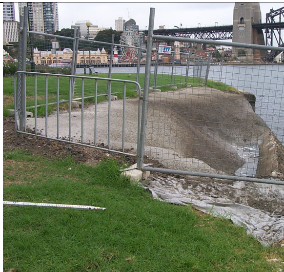
Seawall reconstruction at McMahons Point -- before
