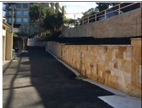
Retaining Wall - Milson Road, Cremorne - After
