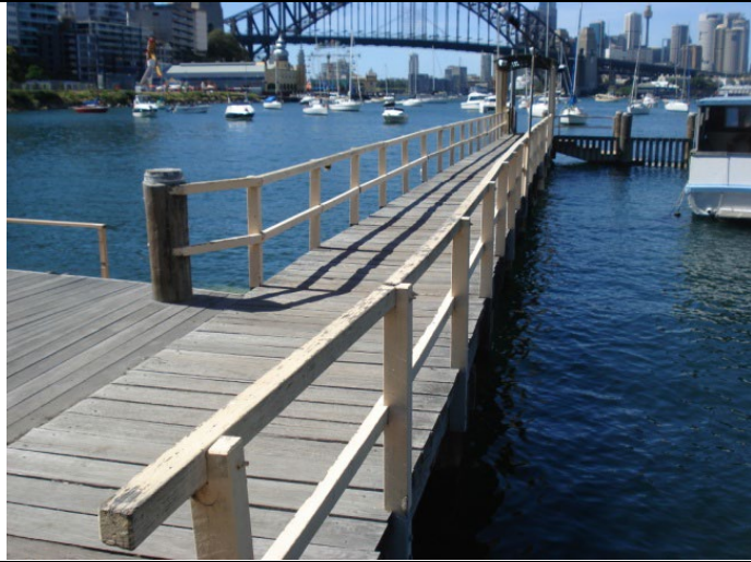
Marine Structures - Lavender Bay Jetty - before
