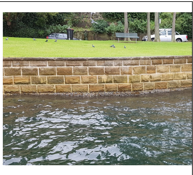
Seawall reconstruction at McMahons Point -- after
