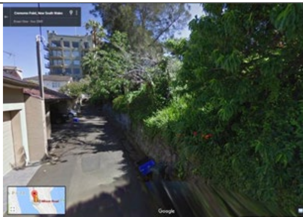
Retaining Wall - Milson Road, Cremorne - Before
