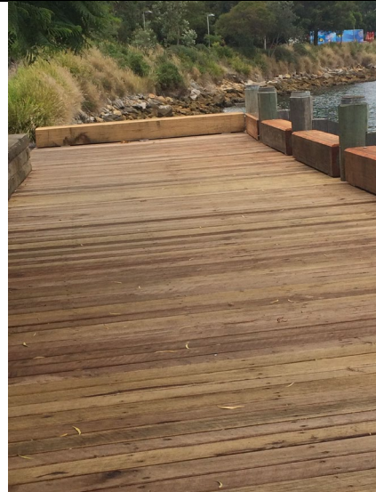
Marine Structures - Lavender Bay Boardwalk - after
