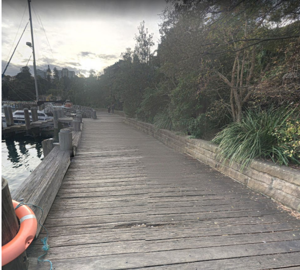
Marine Structures - Lavender Bay Boardwalk - before
