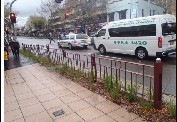
Fences - Military Road Neutral Bay (After) – Decorative Safety Fence
