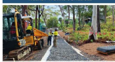
UNDER CONSTRUCTION - FRANCIS DIMOND STREET, ARAKOON
