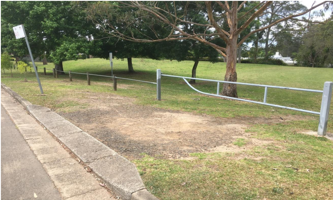
Figures 5,6 Existing Access Points
