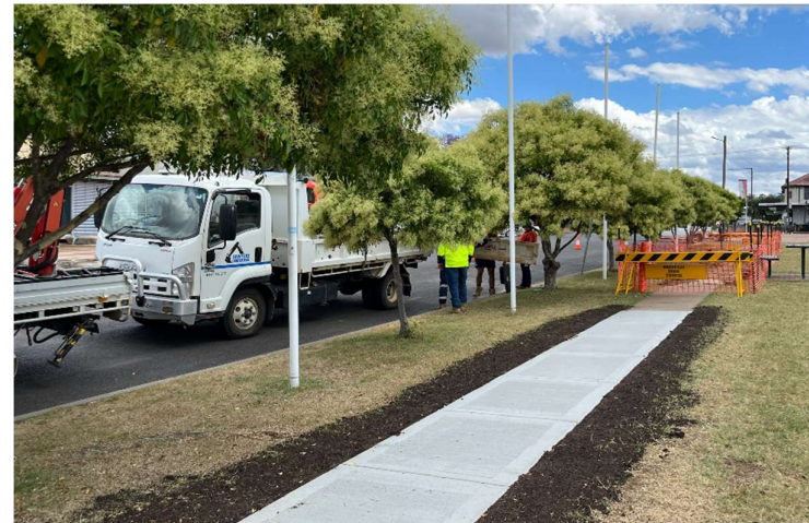
Chandos Street footpath renewal works underway – November 2024
