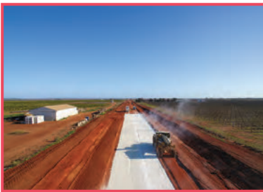
Boorga Road/Dickie Road sealing
