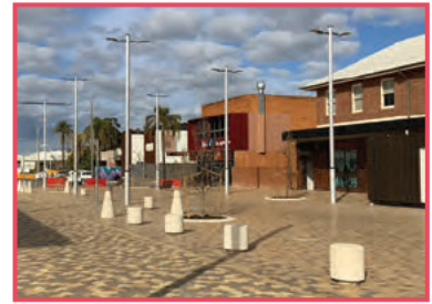
Kooyoo Street redevelopment Stages 1&2
