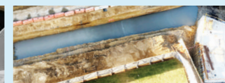
Merrylands Stormwater Upgrade
