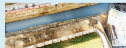
Merrylands Stormwater Upgrade
