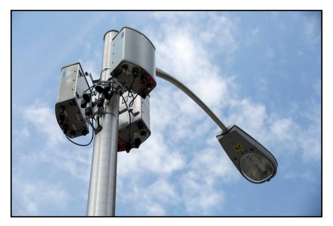
(An example of 5G/Small Cell Equipment mounted on a Light Pole)
