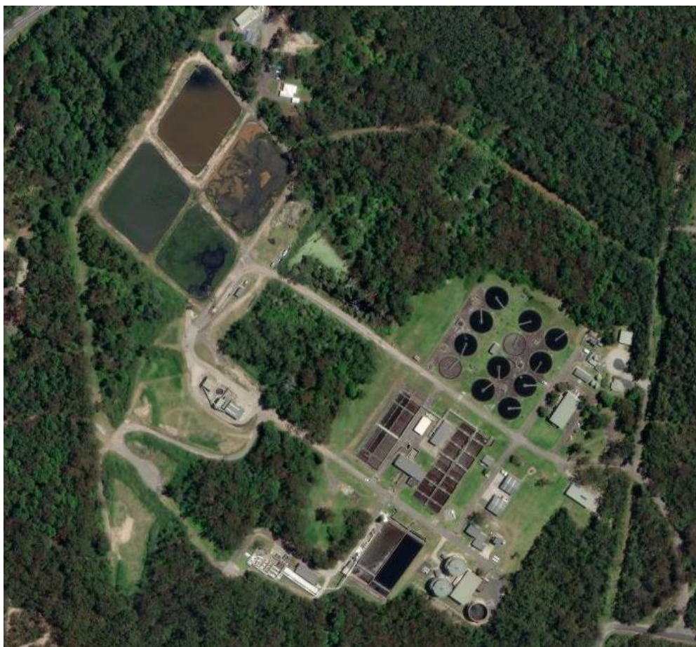
Figure 62: Kincumber STP site overview
