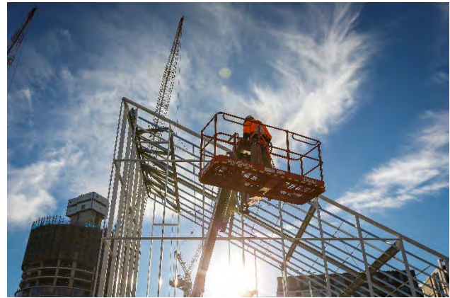
Image 18: Green Square construction work
