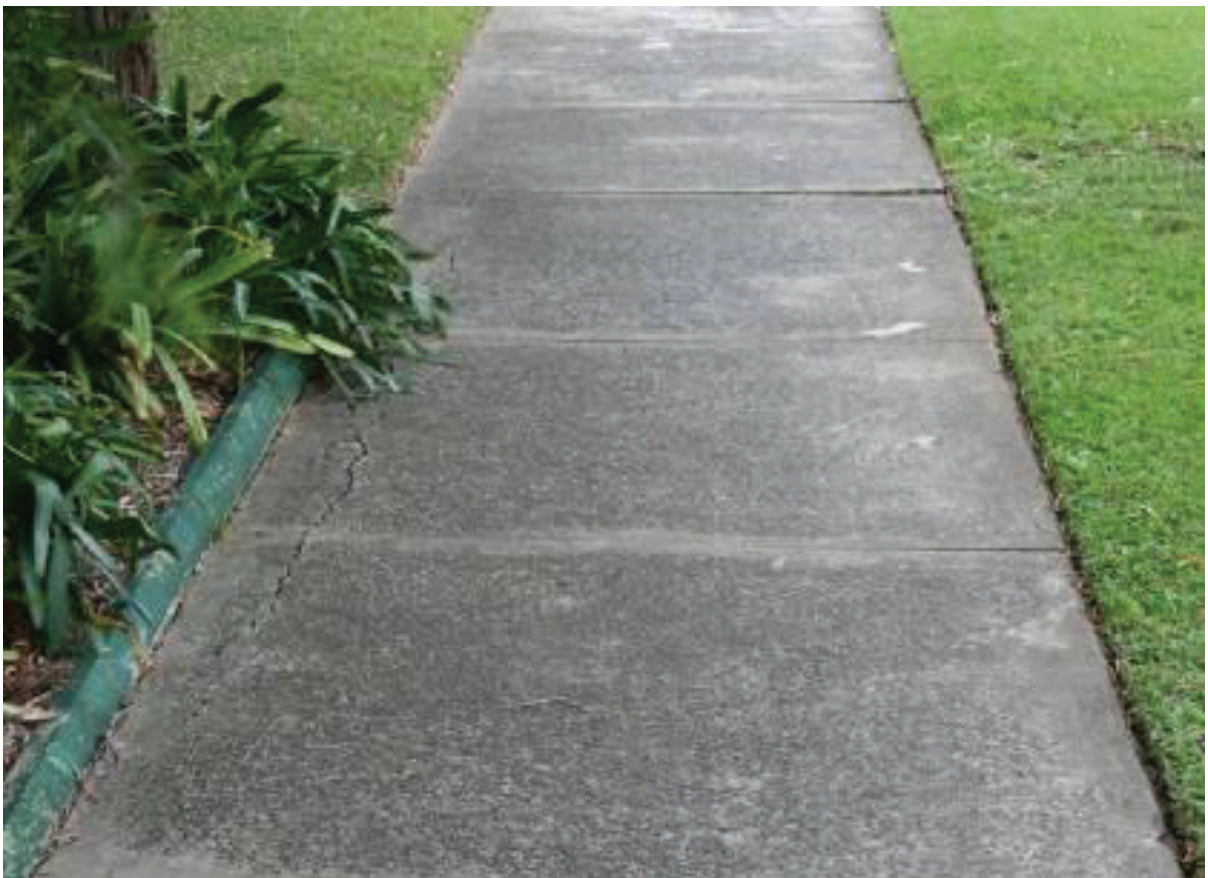
Figure 5 – Example Asphalt Footpath Condition Score 0
