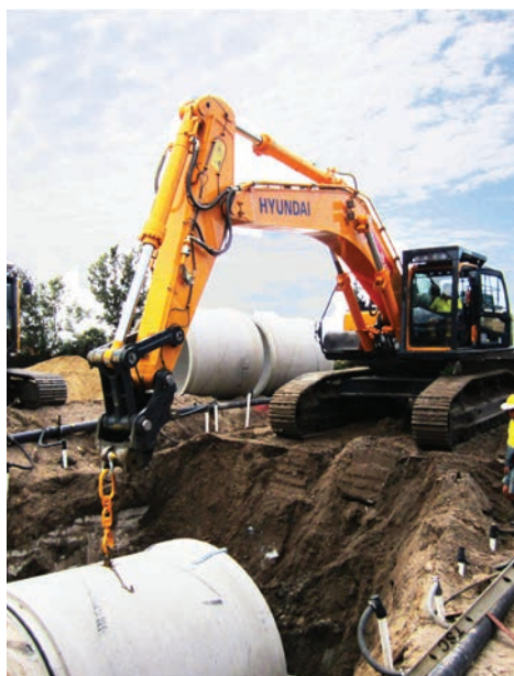
Stormwater pipes being laid at Blue Jay Circuit Kingscliff
