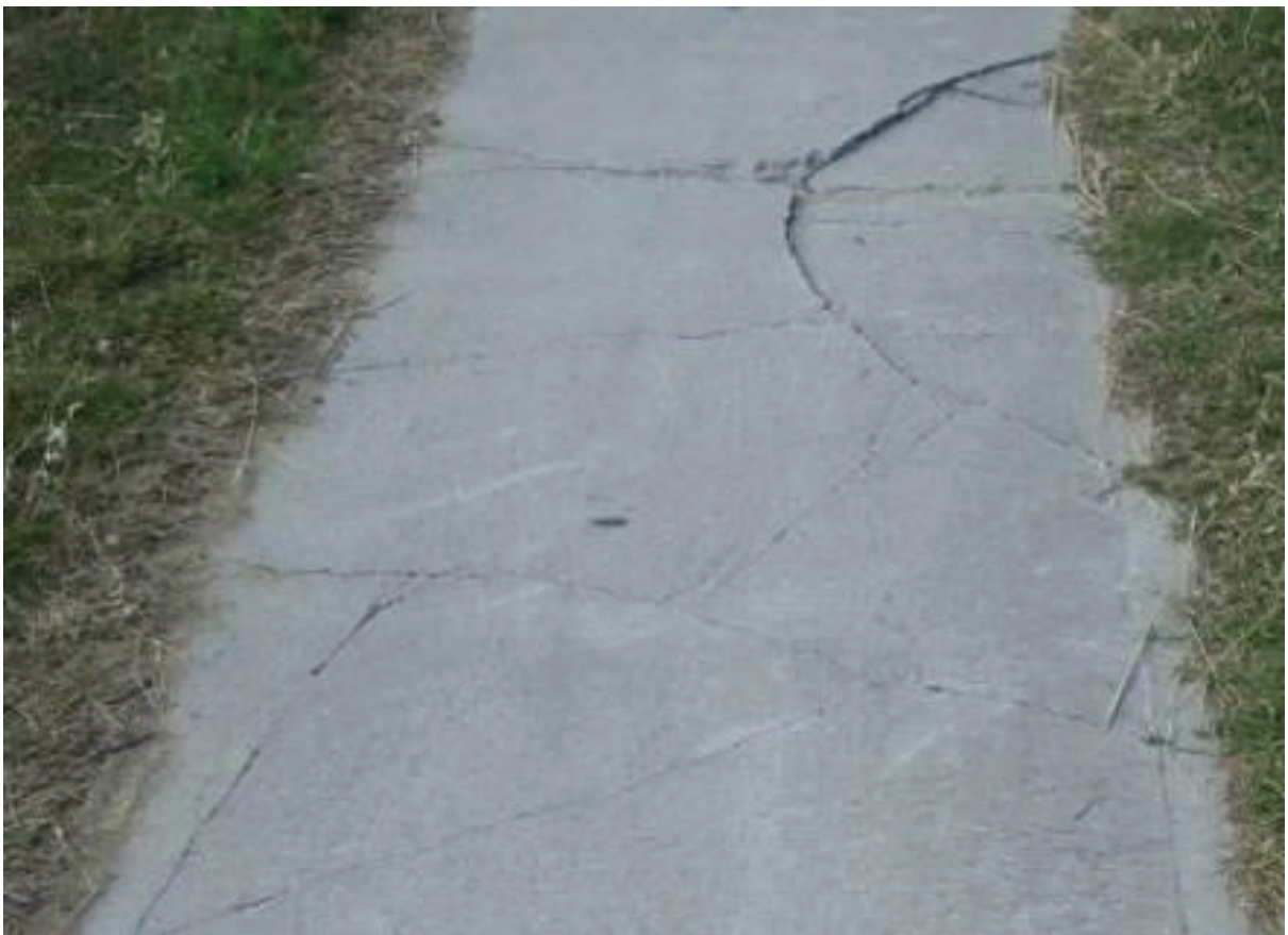
Figure 7 – Example Asphalt Footpath Condition Score 5
