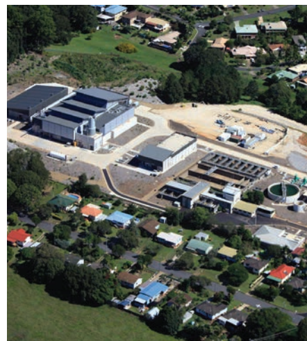
The Bray Park Water Treatment Plant
