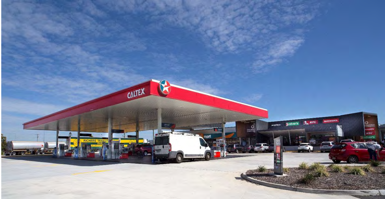
Figure 1 – Northbound Chinderah Service Centre
