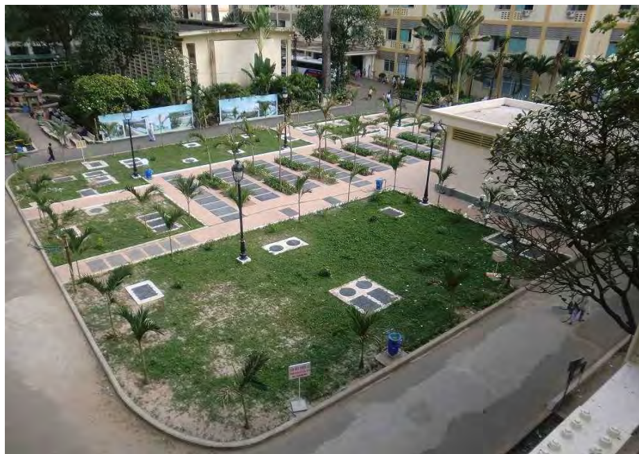
Image 2: Completion of Installation
