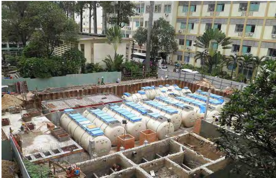
Image 1: Installation of Advanced Sewage Treatment Plant
