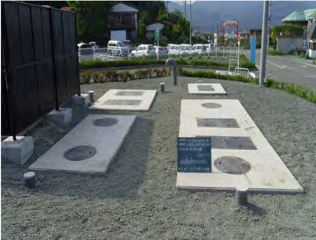
Image 3: Completed Installation of Wastewater Tanks
