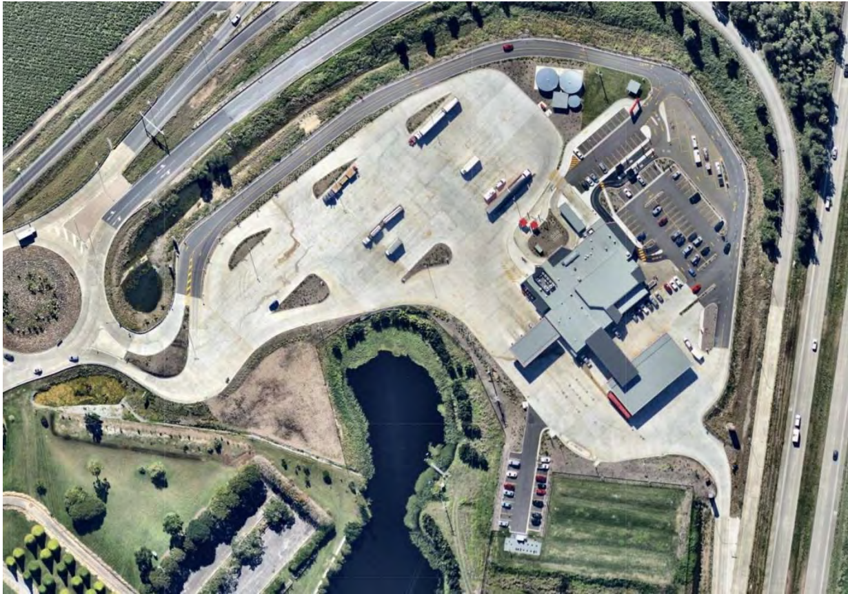
Figure 4 – Aerial View – Chinderah Service Centre (Completion)
