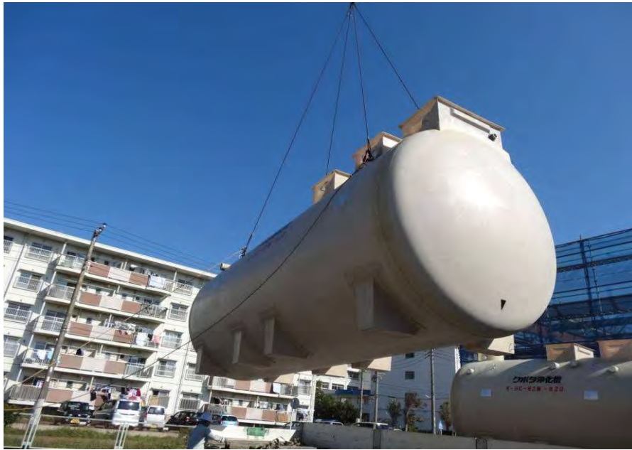
Image 1: Installation of Wastewater Tanks
