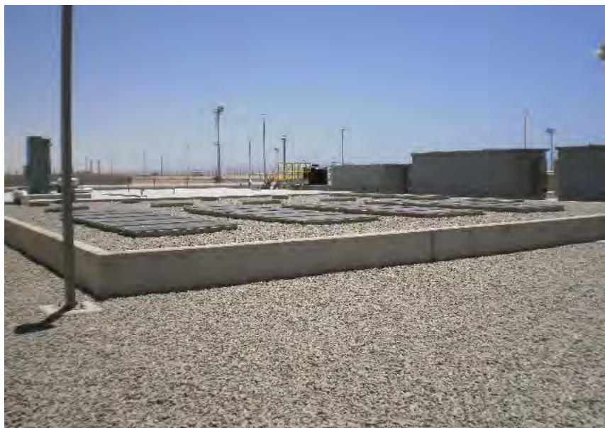
Image 2: Completed Installation of Sewage Tanks
