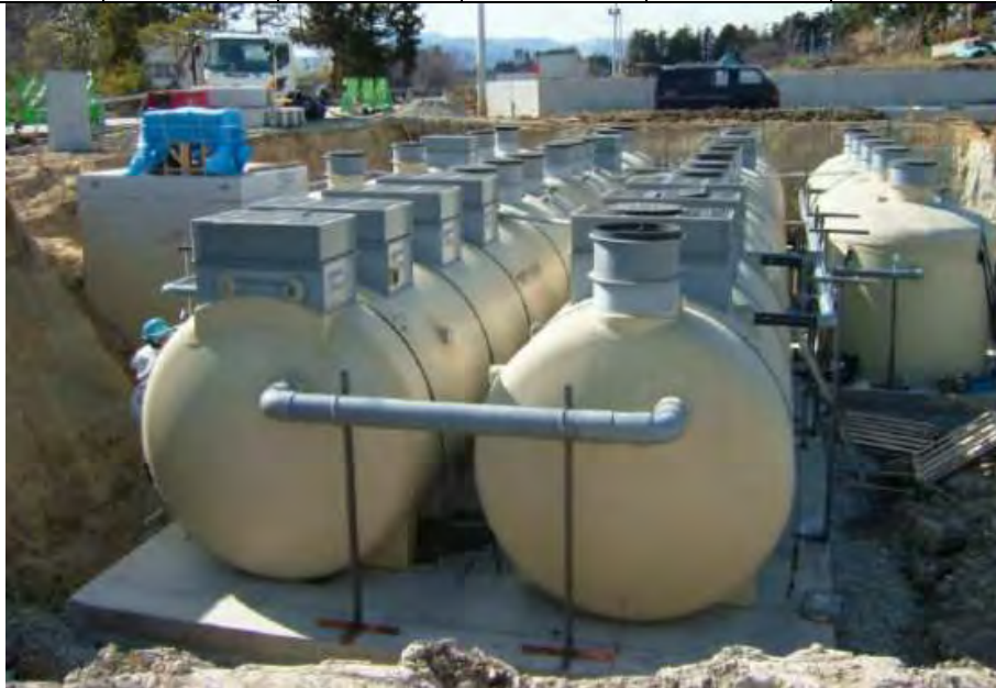
Image 1: Installation of Advanced Sewage Treatment Plant
