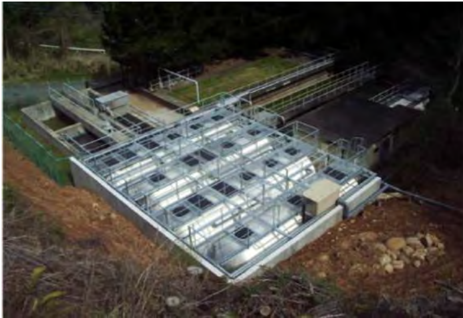
Image 1: Installation of Advanced Sewage Treatment Plant
