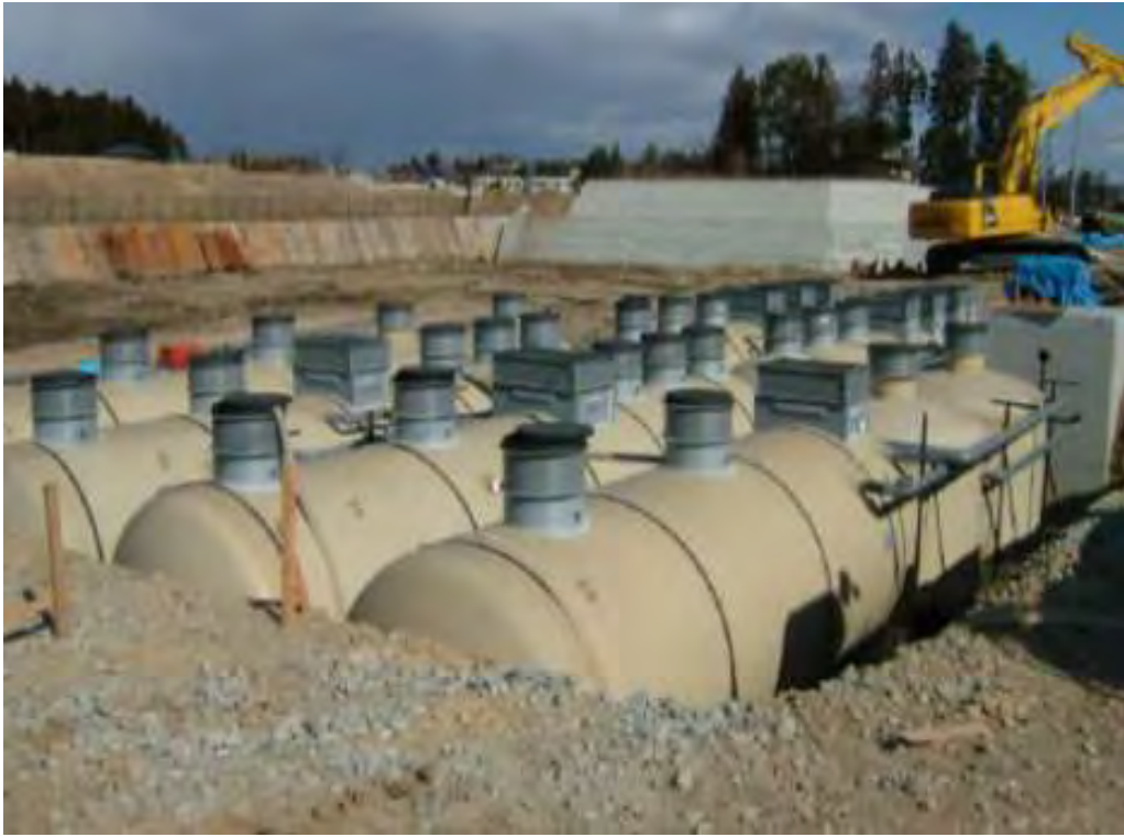
Image 3: Tank Configuration for Sewage Treatment Plant
