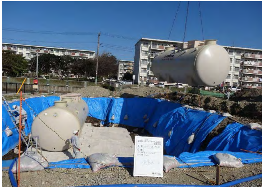
Image 2: Installation of Wastewater Tanks Continued
