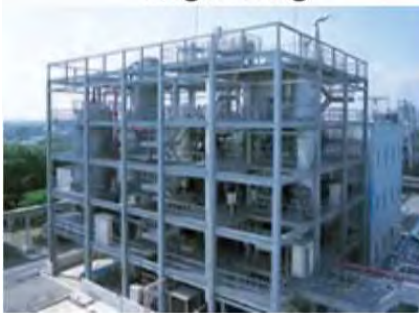
Sludge Treatment Plant
