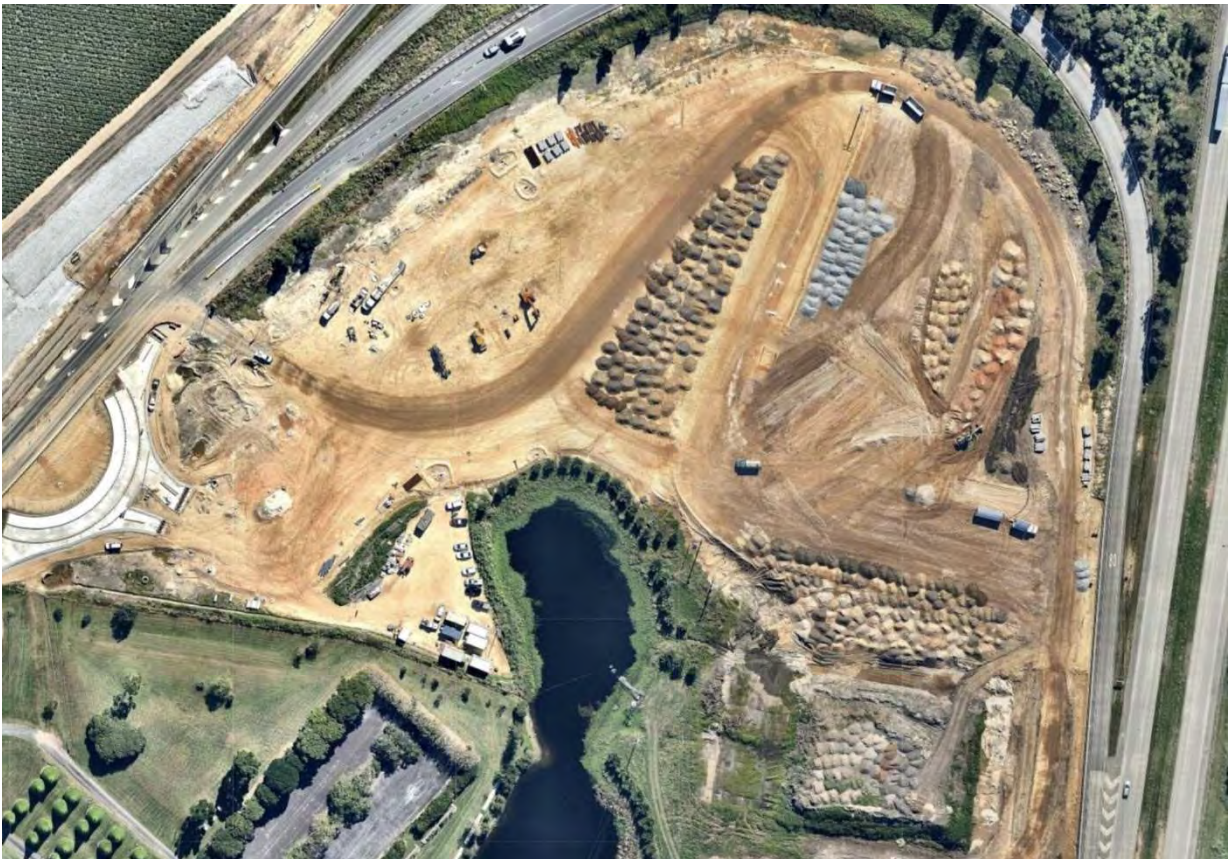
Figure 3 – Aerial View – Chinderah Service Centre (During Civil Construction)
