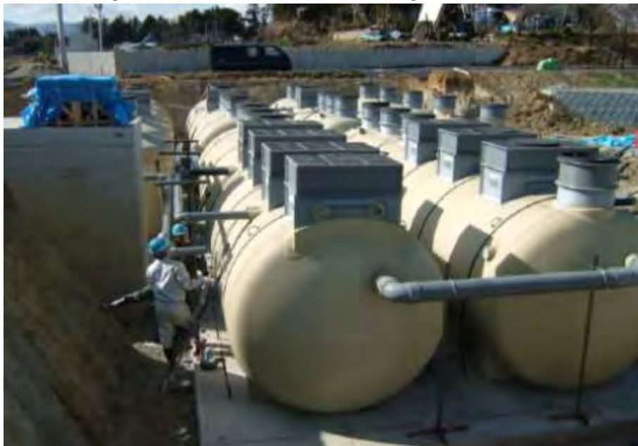
Image 2: Installation of Advanced Sewage Treatment Plant
