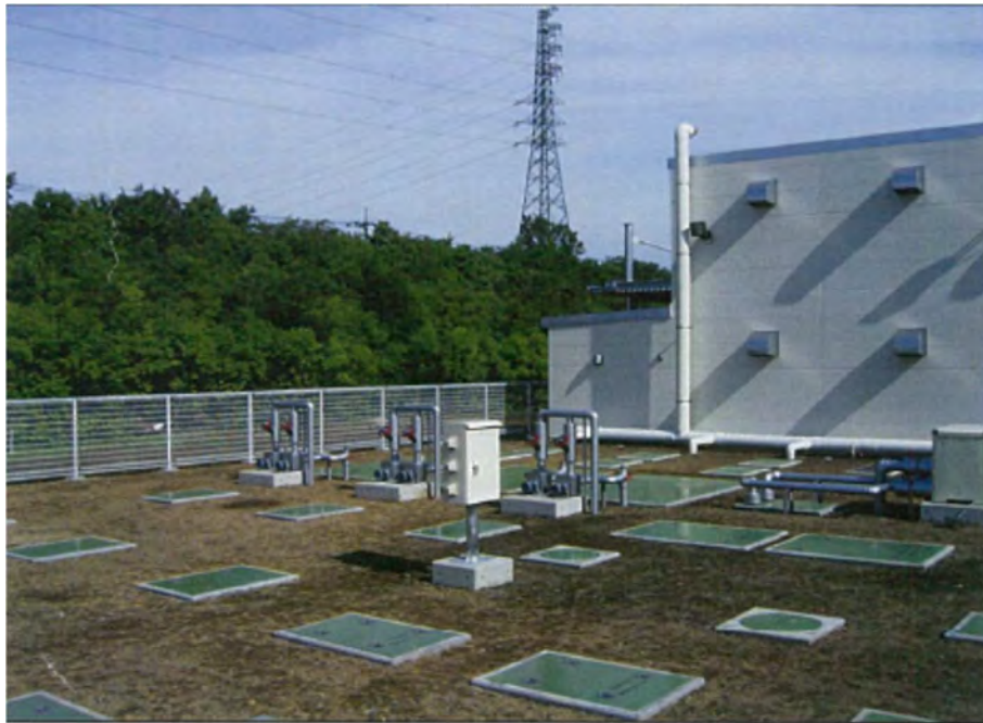
Image 1: Completed Installation of Treatment Tanks
