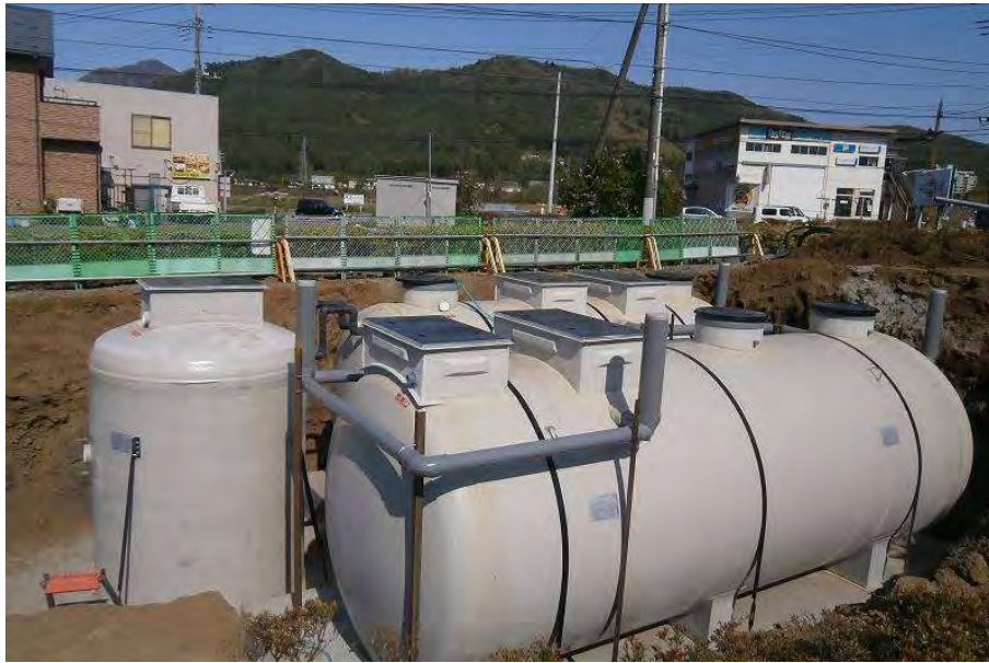
Image 1: Installation of Wastewater Tanks
