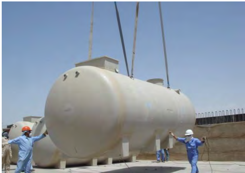
Image 1: Installation of Advanced Sewage Treatment Plant
