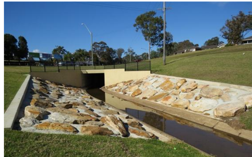
(Culvert extension work, Bradbury Park)
