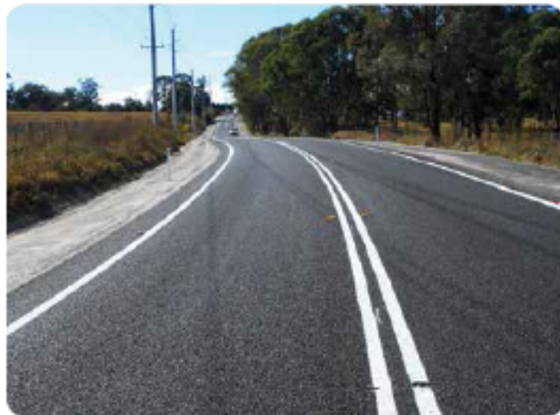
The upgraded section of King Road at Ribberoonce. The SRV would help Council to maintain and upgrade roads that would meet community expectations.
