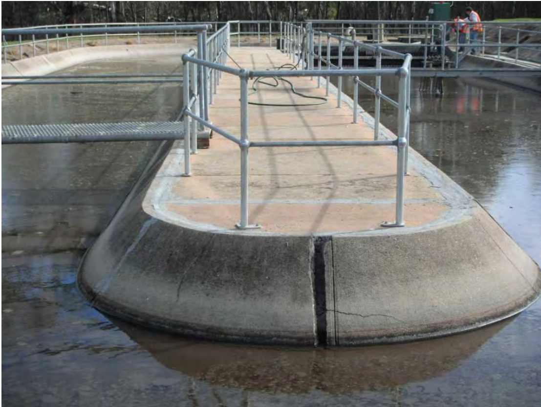
Figure 4: Corroded and non-compliant walkways, Holbrook STP (safety)
