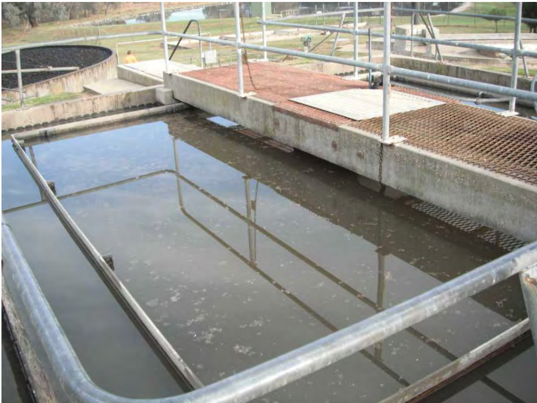
Figure 4: Corroded and non-compliant walkways, Holbrook STP (safety)
