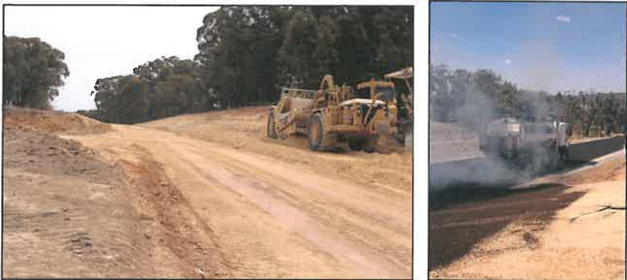
Taralga Road MR248E construction
