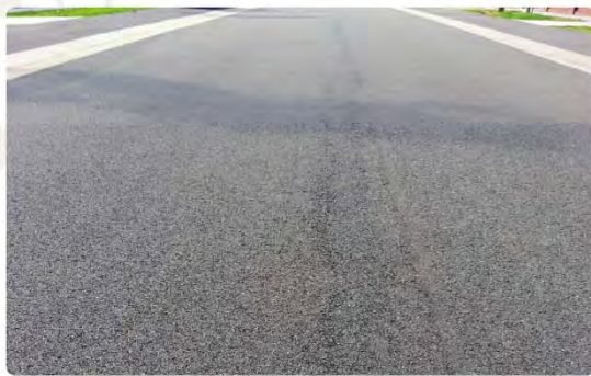
Condition 1 - Byron Street, Croydon
