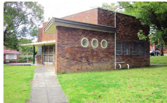
Condition 5 - YMCA Building Yeo Park
