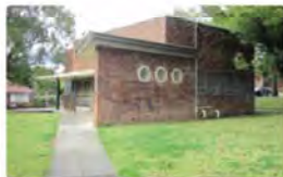
Condition 5 - YMCA Building Yeo Park
