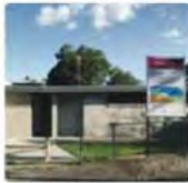
Pratten Park change rooms
