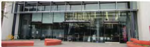
Condition 1 - Ashfield Civic Centre
