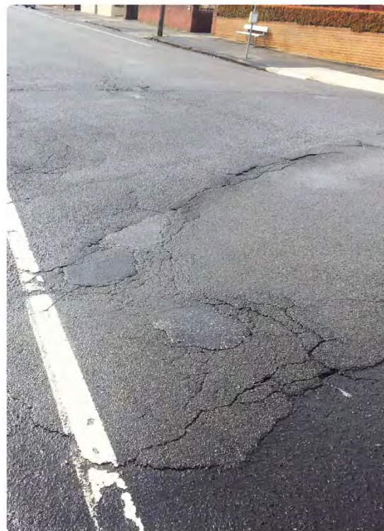
Condition 5 - Dalhousie Street, Haberfield
