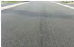
Condition 1 - Byron Street, Croydon
