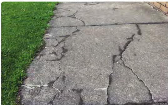
Condition 4 - Seaview Street, Summer Hill
