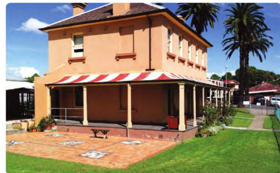
Condition 3 - Thirring Villa Pratten Park
