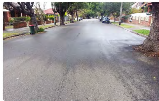
Condition 2 - Denman Street, Haberfield
