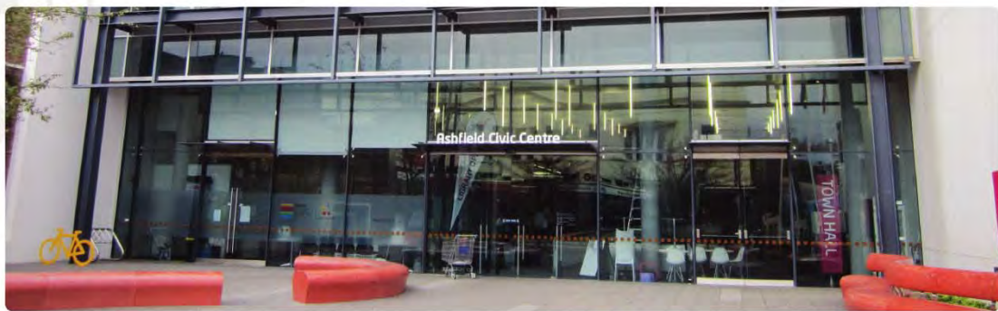
Condition 1 - Ashfield Civic Centre
