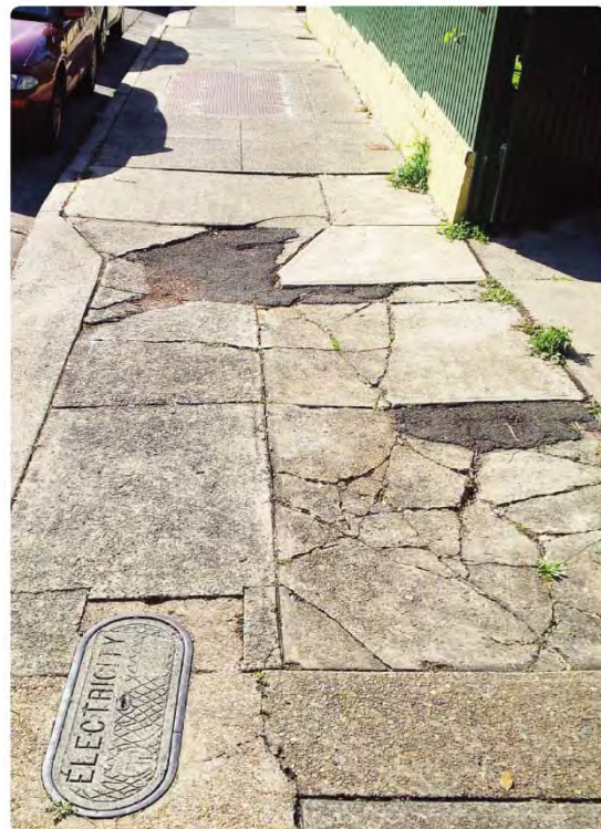
Condition 5 - Bland Street, Ashfield
