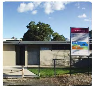
Pratten Park change rooms
