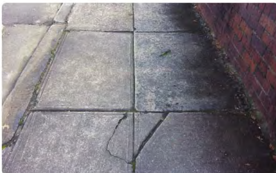
Condition 3 - Arthur Street, Ashfield
