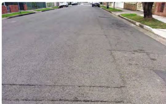
Condition 3 - Carshalton Street, Croydon
