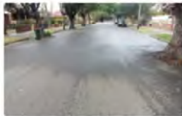
Condition 2 - Denman Street, Haberfield
