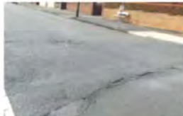
Condition 5 - Dalhousie Street, Haberfield
