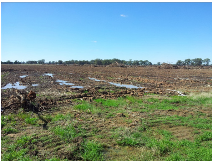
Below: Ground cleared and ploughed
