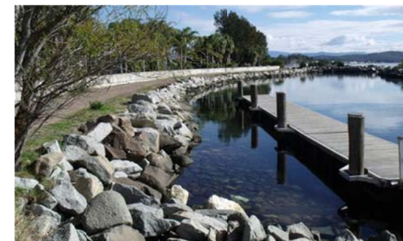
Hanging Rock Pontoon
