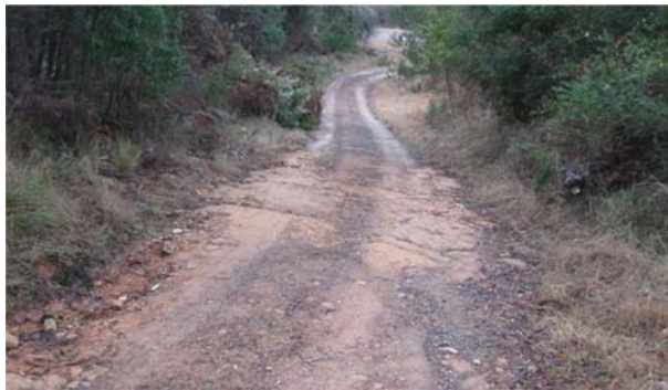
An Increase in rural road resheeting (pictured a road in need of resheeting)
