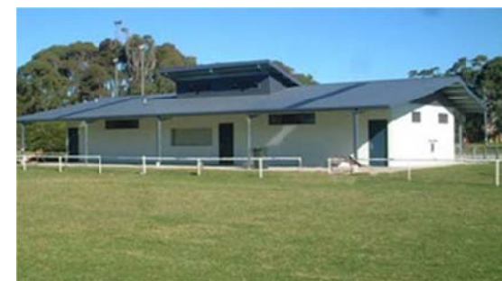
Bill Smyth Oval amenities building renewed in 2007
