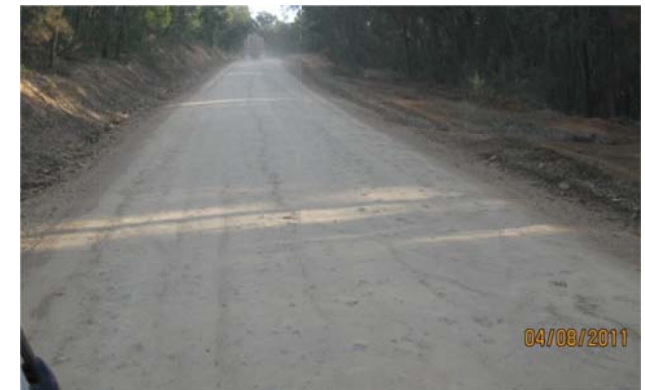
Araluen Road before & after resheeting
