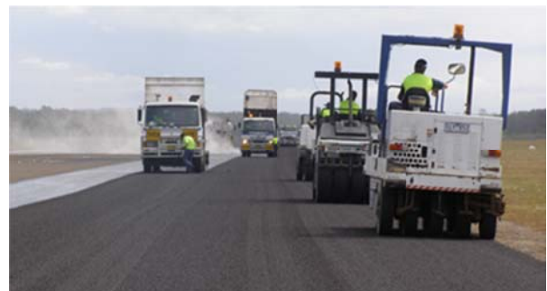
Resealing roads is vital to protecting the underlying pavement of the road network, council has focused resources toward reseals (a reseat of the airport runway pictured above)
