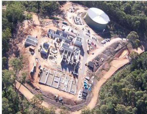
Northern Water Treatment Plant
