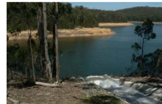
New pipeline delivers water into Deep Creek Dam
