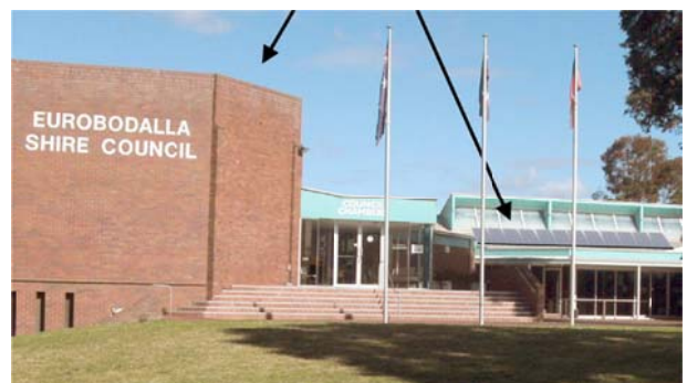
New solar panels have been identified for installation on the administration building as part of a planned energy efficiency program, savings are already being achieved at Moruya and Batemans Bay Pool
