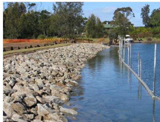
Tomago River Estuary rockwall protection works undertaken
