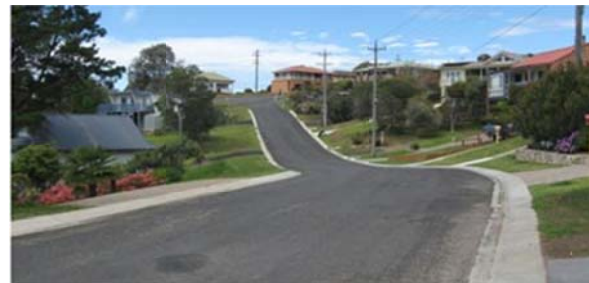
Urban Roads Reconstruction Program (above images show before & after reconstruction of Hadrill Parade, Dalmeny)
