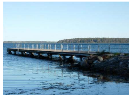
Jetty in "good" condition
