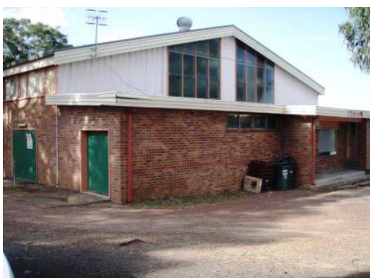
Building in "fair" condition
