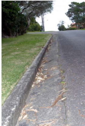
Kerb and Gutter in "fair" condition
