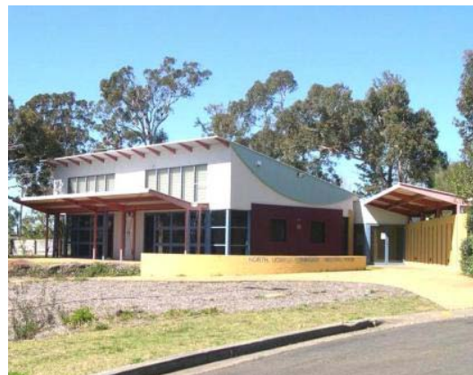
Building in "good" condition
