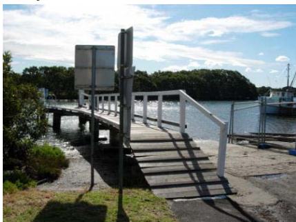
Jetty in "fair" condition
