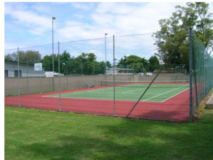
Recreational facility in "good" condition
