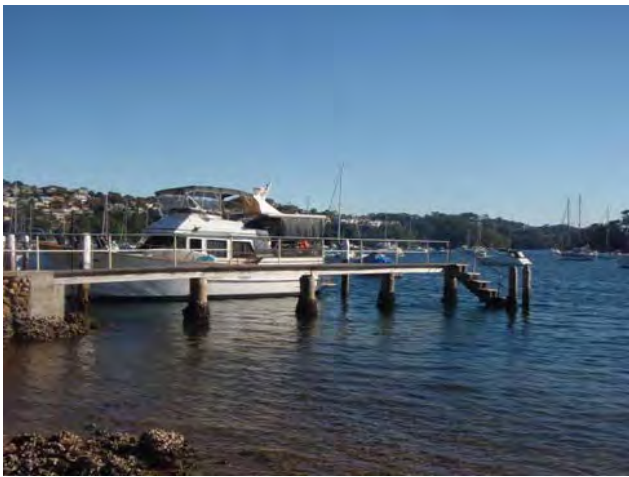
Figure 3: Inkerman Street Jetty
