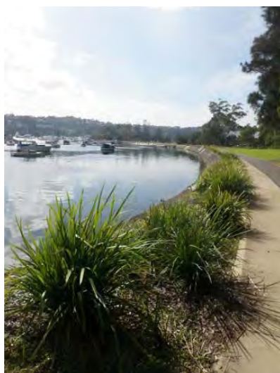
Figure 5: Concrete Seawall - The Spit - RW79
