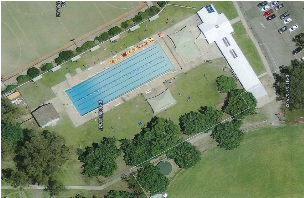
Figure 3 Corowa Swim Centre Aerial
